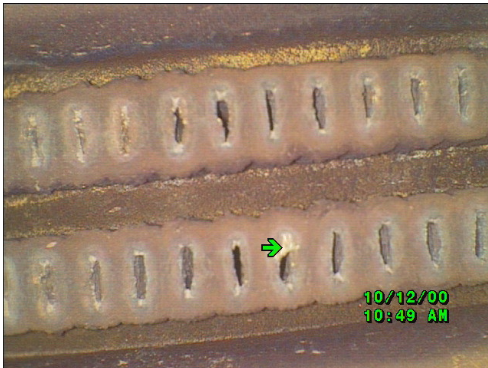
Figure 2: Hollow Conductors with Copper Oxide Plugging at the Water Inlet End [9].
